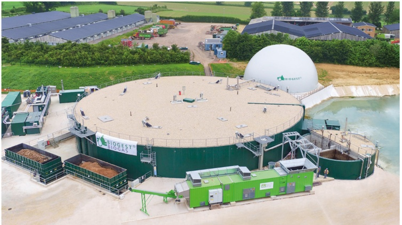
PowerRing Biomethaneinspeiseanlage Frogmary in UK
